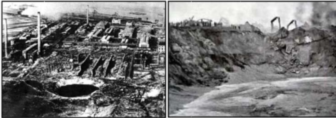
Figure 1 - The consequences of explosion caused by blasting of hardened fertiliser, Opau, Germany, 1921 (French Ministry of Sustainable Development, 2008)
